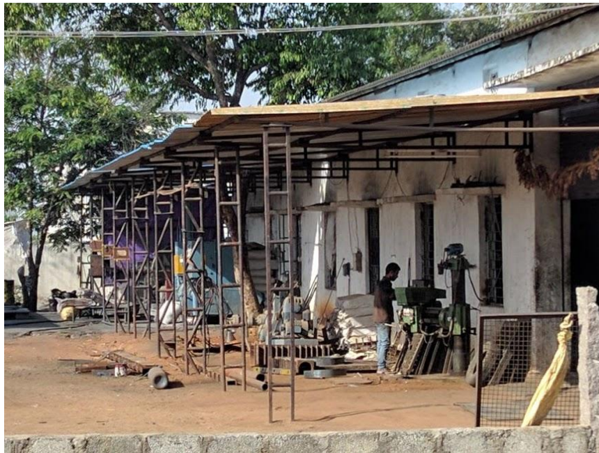
Welding & Gas Cutting Area
